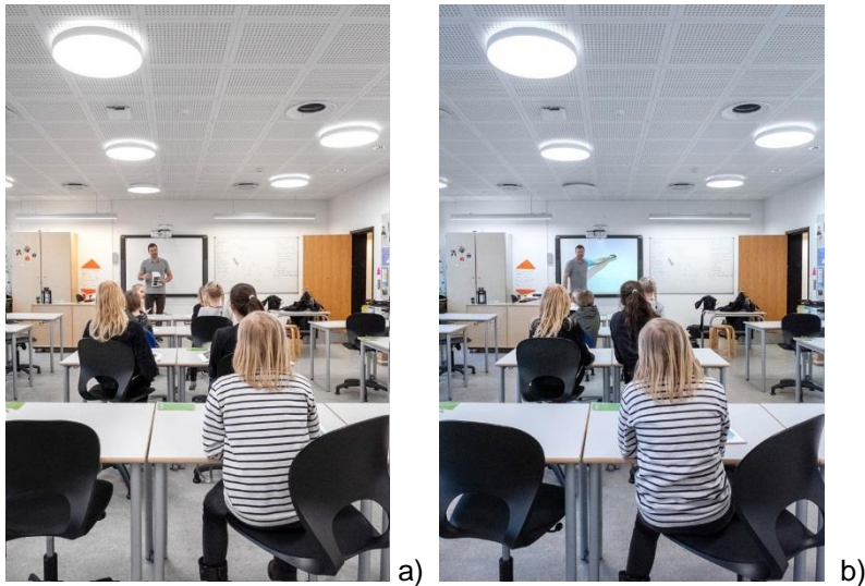
Fig. 1a (3000K), b (6000K): After half an hour, the smart board is switched on. The teacher adjusts the light settings to help students concentrating on the smartboard. At the same time, good visibility of exercise books and materials at the student workspaces remains unaffected.
